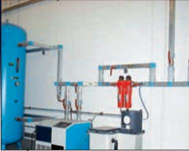
Distribution pipework in aluminium for compressed air, vacuum and other non dangerous gases, from 20 to 110 mm diameter.
