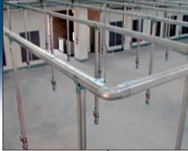
Drops to the point of use, fast and easy to assemble or modify.
